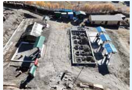
Underground Fuel Storage Tanks
