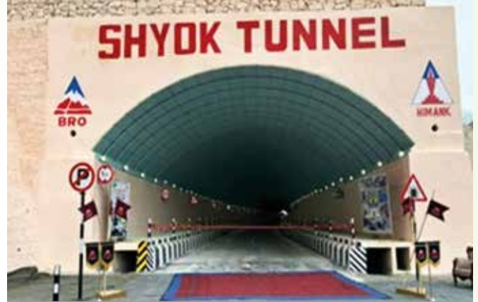
SHYOK TUNNEL Connecting : Darbuk- Shyok- Daulat Beg Oldie
