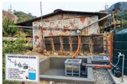
Rain Water Harvesting Capacity 1000 - 50,000 L Size 1-2.5 m dia tanks
