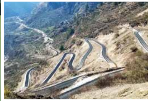
Forward connectivity (Above : Ghatiabagarh - Lipulekh Road)
