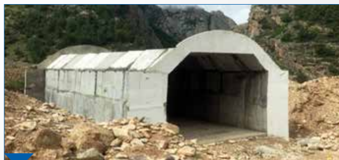
Force Preservation Bunker
